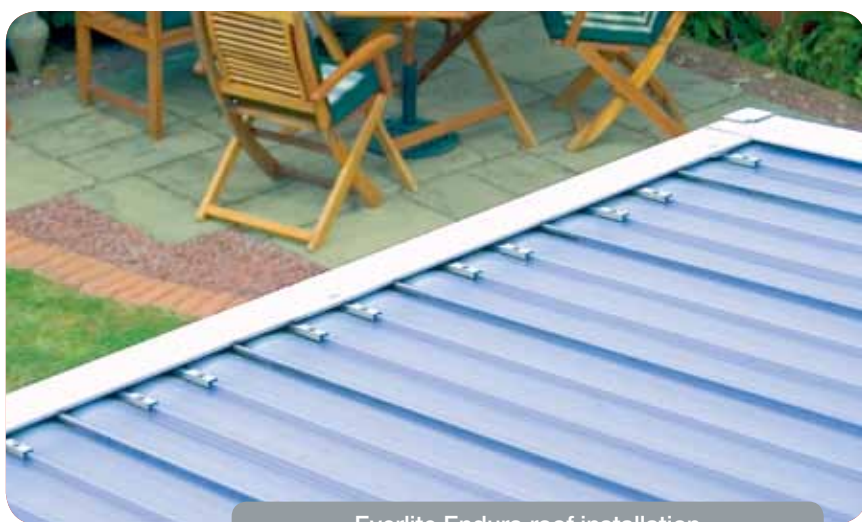
Everlite Enduro roof installation
