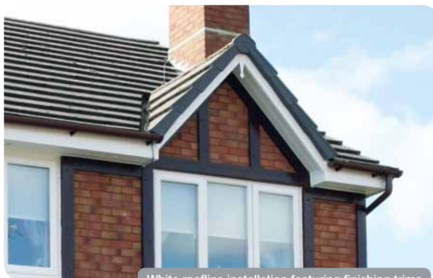
White roofline installation featuring finishing trims
