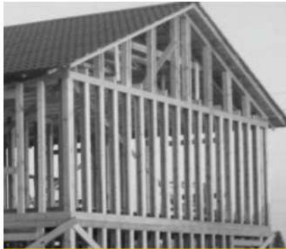
Timber frame construction
