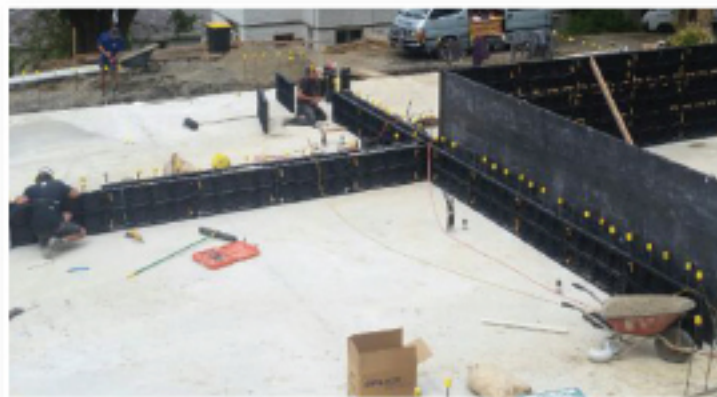
Formwork set up
