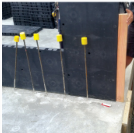
Formwork set up
