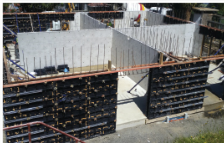
Cross Wall formwork
